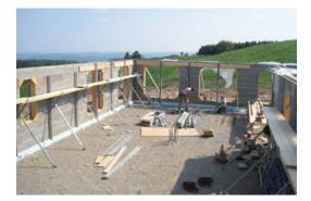
everything else was designed around that: the shape and size of the walls were designed to make use of full blocks with no need for cutting or re-shaping.
