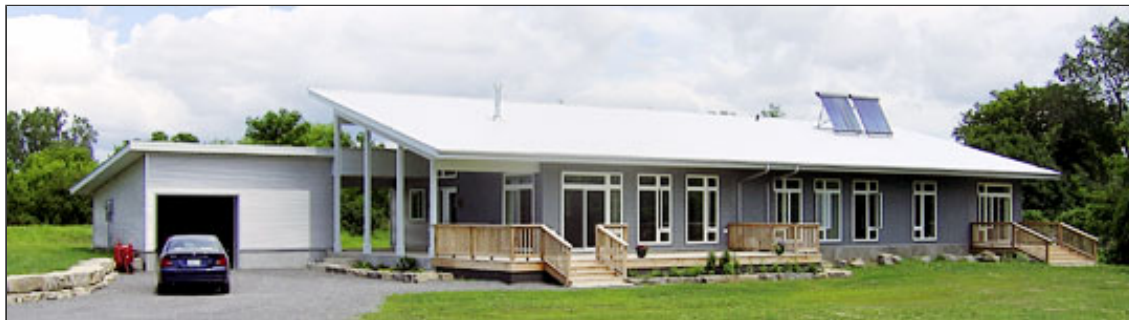
The completed County Trail House, like all Solares homes, features passive solar design.
